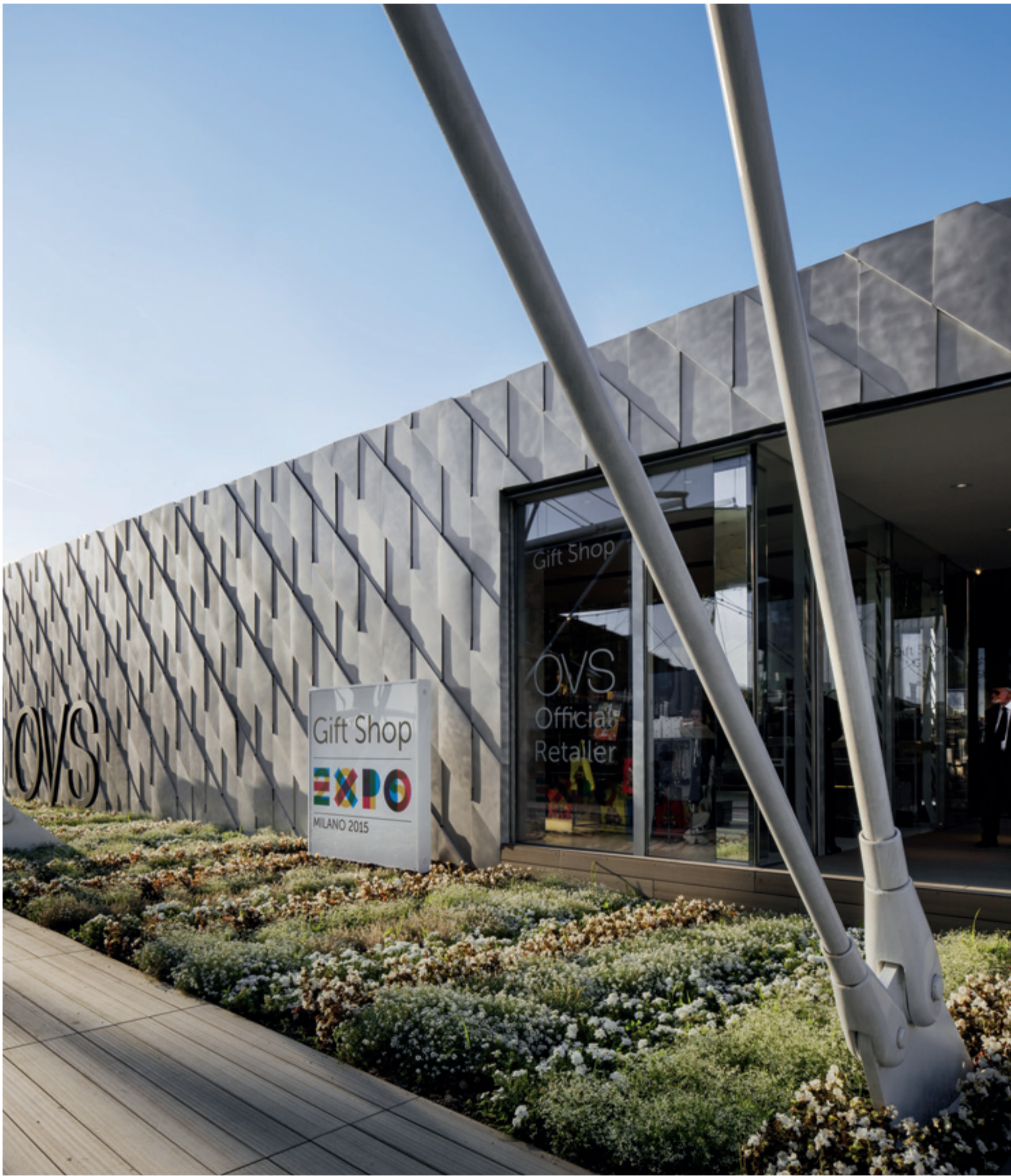
"OVS PAVILIONS", 2015 Rivestimento in alluminio spazzolato / Brushed aluminium wall covering
